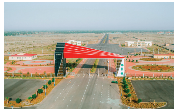
The gates of the Bulbula Integrated Agro-Industrial Park
